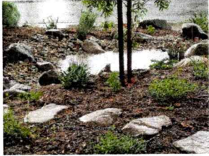
Stone lining the ponding zone of this rain garden. Image credit California Native Plant Society ( https://www.flickr.com/photos/152508454@N05/ )
