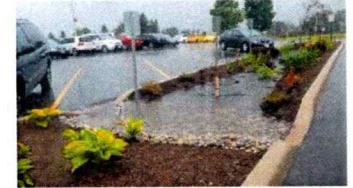
This bioswale in a parking lot uses stone at the inlets and along the bottom of the swale to prevent erosion, as the sides are sloped.
